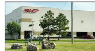
SWEF facility in Tulsa, OK
