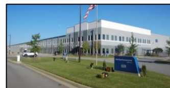
CO 2 systems plant in Conyers, GA
